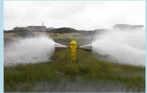
Flushing A Water Main
